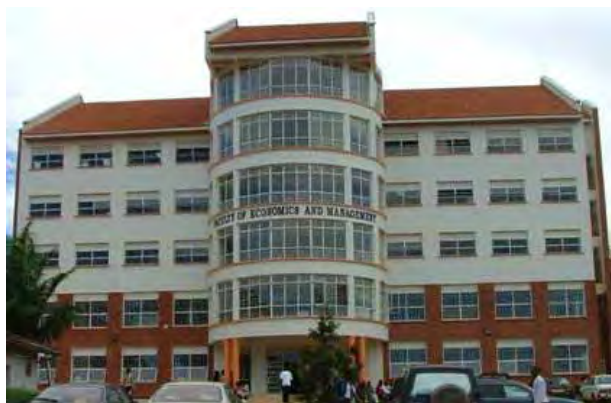
Faculty of Economics and Management One of the new buildings from Internally generated fund (one floor was contributed by the ACBF)
